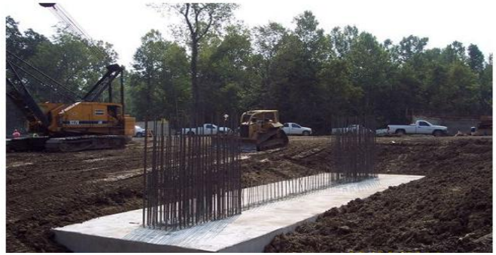
Figure 2.5 Construction of a combined footing
